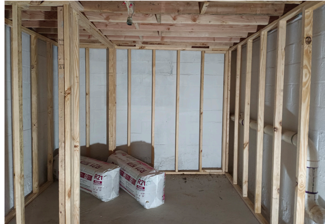
1. BASEMENT ADDITION - LOOKING NORTH
