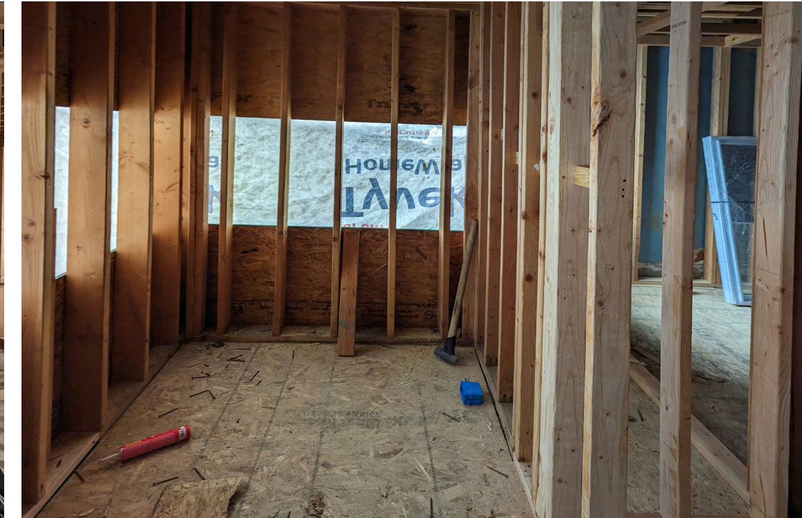
4. 2ND FLOOR ADDITION - LOOKING EAST
