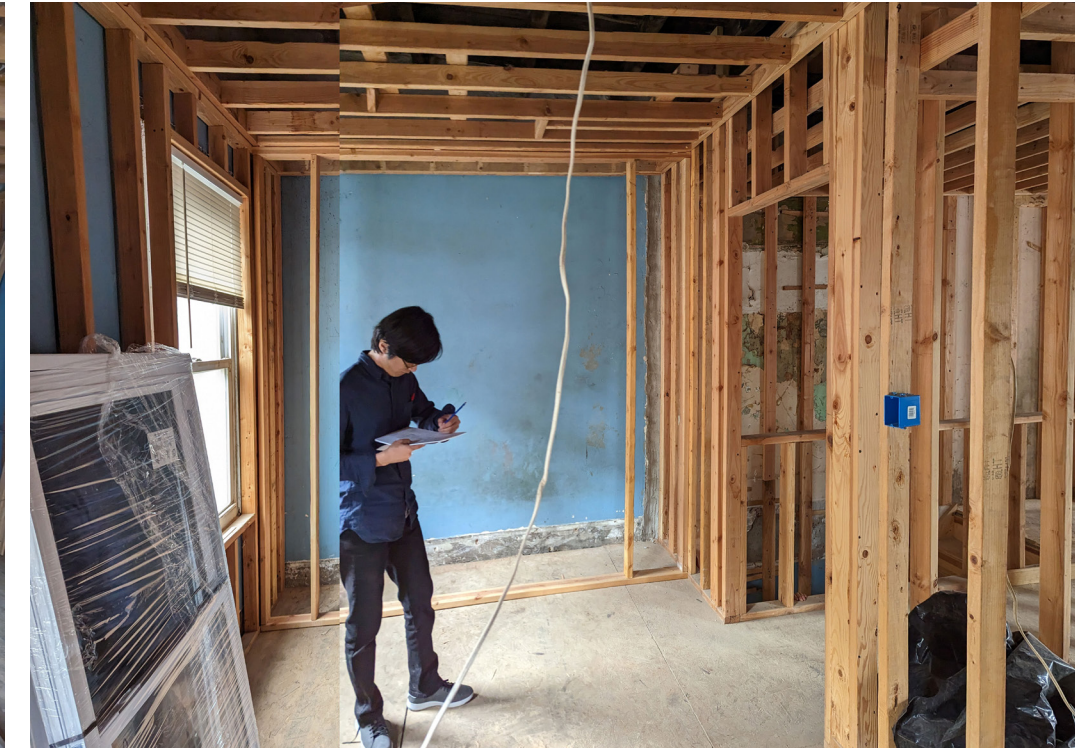
3. 2ND FLOOR SOUTHSIDE ROOM LOOKING WEST
