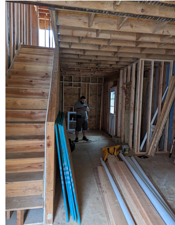
2. 1ST FLOOR FROM FRONT ENTRANCE
