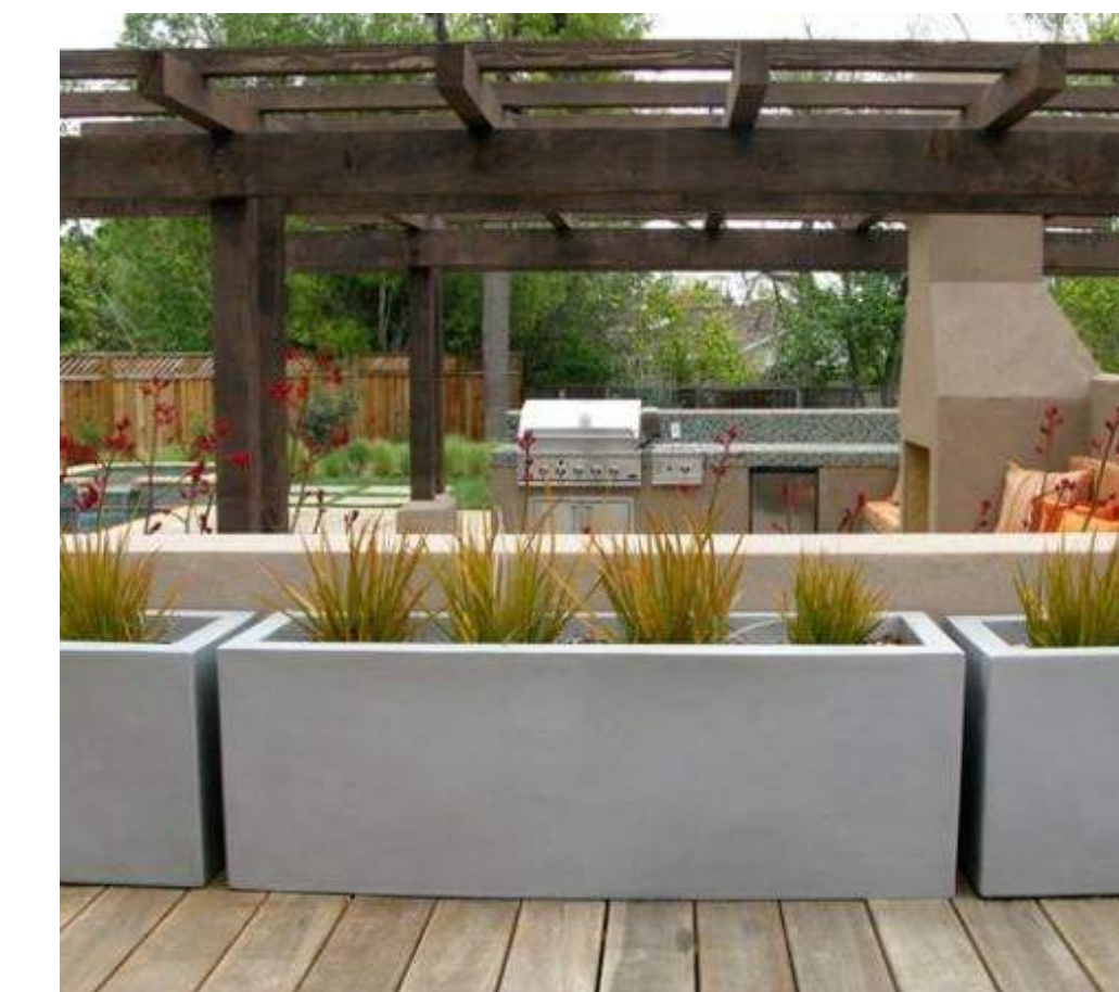
9- Cast in Place Concrete Planter Box- Smooth
