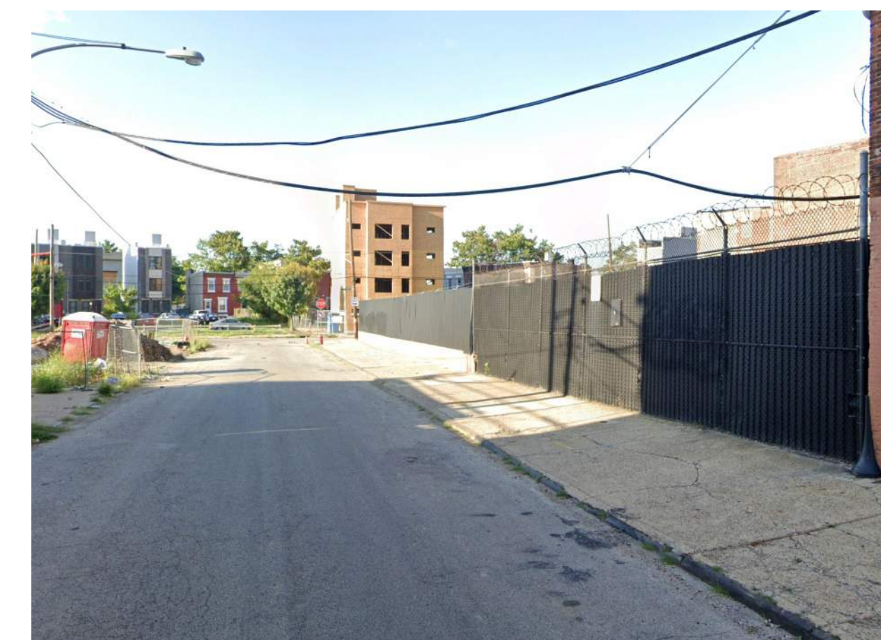
3 - VIEW ON RANDOLPH STREET LOOKING NORTH
